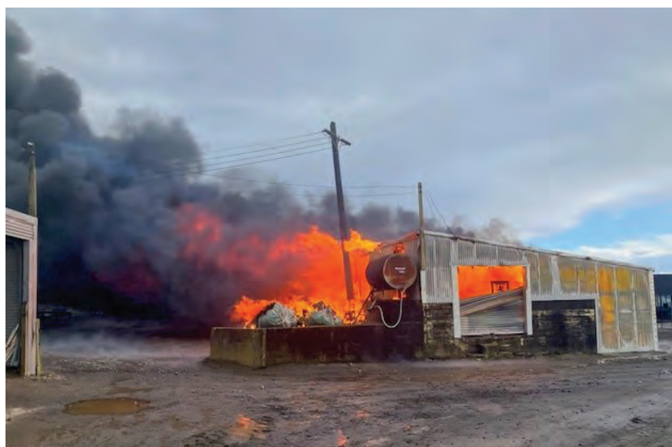
Within a short time a workshop and storage shed went up in flames...
